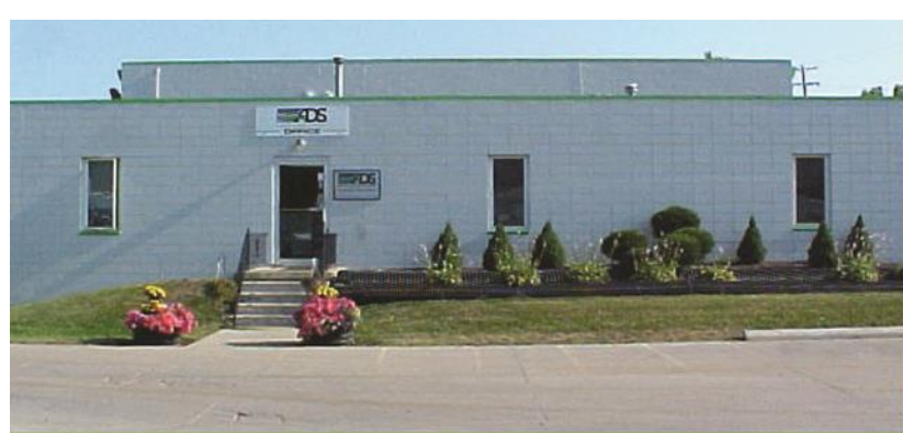
Owosso Manufacturing Facility
