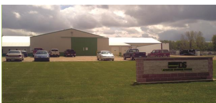
Clifford Manufacturing Facility
