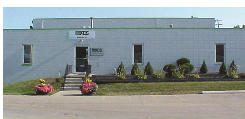
Owosso Manufacturing Facility
