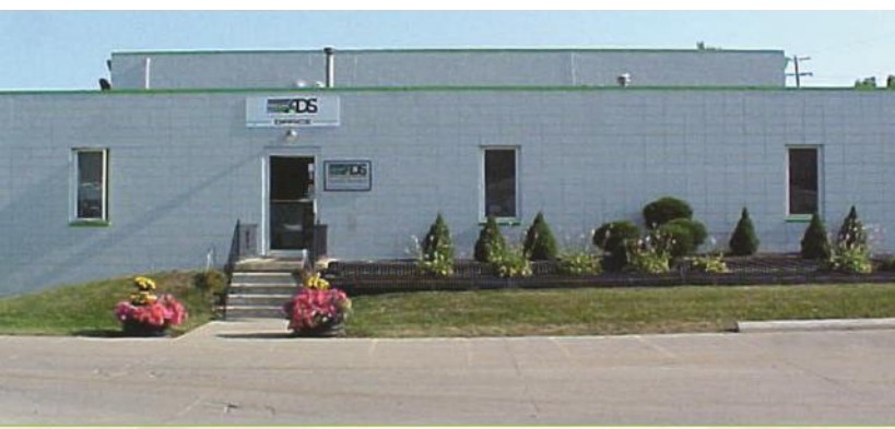
Owosso Manufacturing Facility
