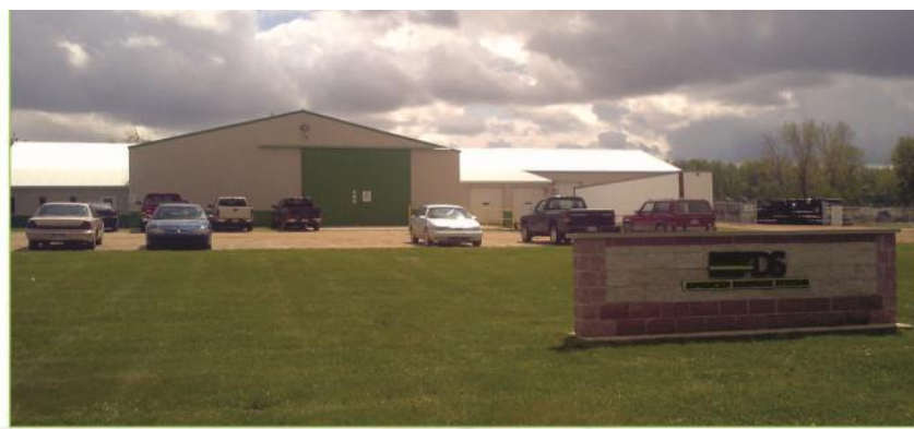
Clifford Manufacturing Facility
