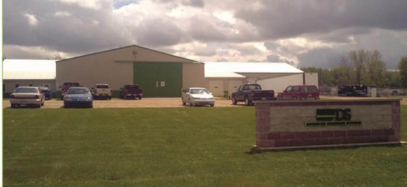
Clifford Manufacturing Facility
