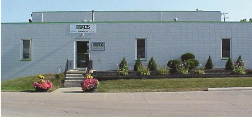
Owosso Manufacturing Facility
