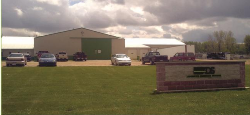
Clifford Manufacturing Facility
