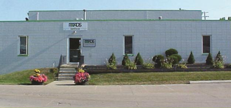
Owosso Manufacturing Facility
