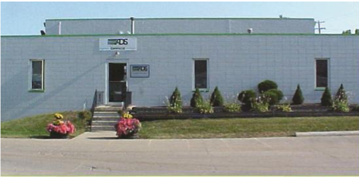
Owosso Manufacturing Facility
