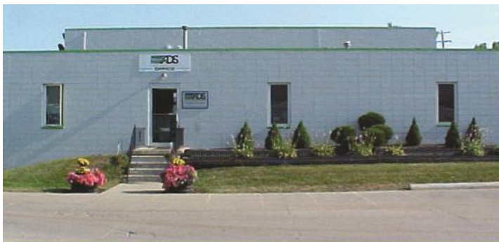
Owosso Manufacturing Facility
