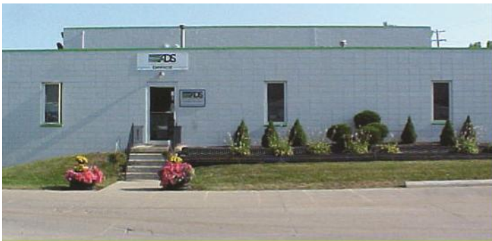
Owosso Manufacturing Facility
