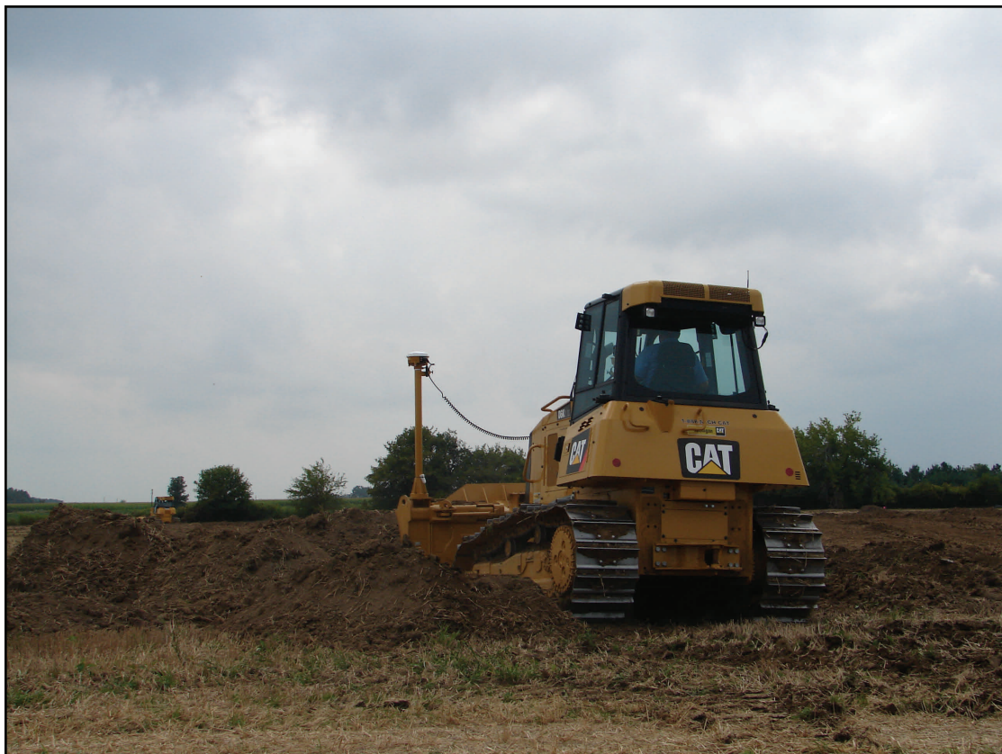
CAT Dozer doing some land shaping work at 2014 Field Day. Thanks to Michigan CAT for bringing a couple of them up for contractors to try out.
